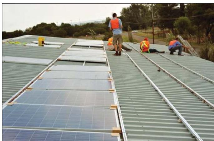
Fig. 6: 15 kW PV grid tied system.
