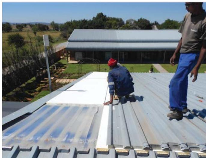
Fig. 5: Roof insulation installation.
